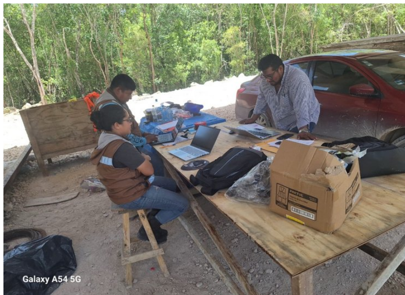
On-site technical and administrative control.
