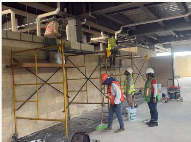
05 • Masonry and partitions
