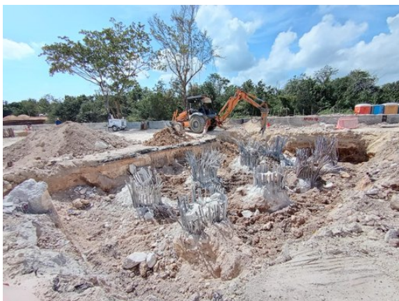
Earthmoving at the work front.
